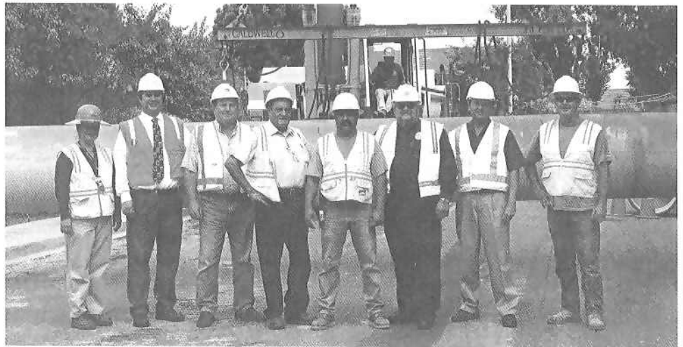
Representatives from OWD and Ortiz Construction prepared to install the final section of 30-inch in diameter pipe as the project nears completion.
